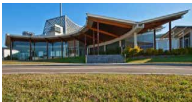
Fot. 4 OPAL – Open Pool Australian Light Water Reactor (fot. ANSTO z prezentacji Jason Chakovski & Andrew Frikken) Photo. 4. OPAL – Open Pool Australian Light Water Reactor
