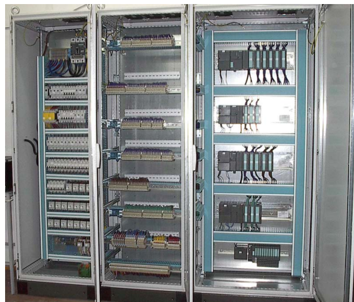
Fig. 15. Control panel with fuse and breaker unit, connection unit, and microprocessor and interface module units
