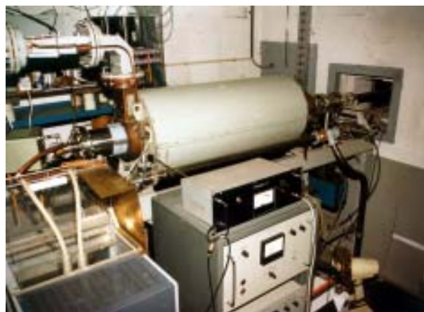
Fig. 1. General view of the linear electron accelerator (LAE 10) installed in the INCT.
